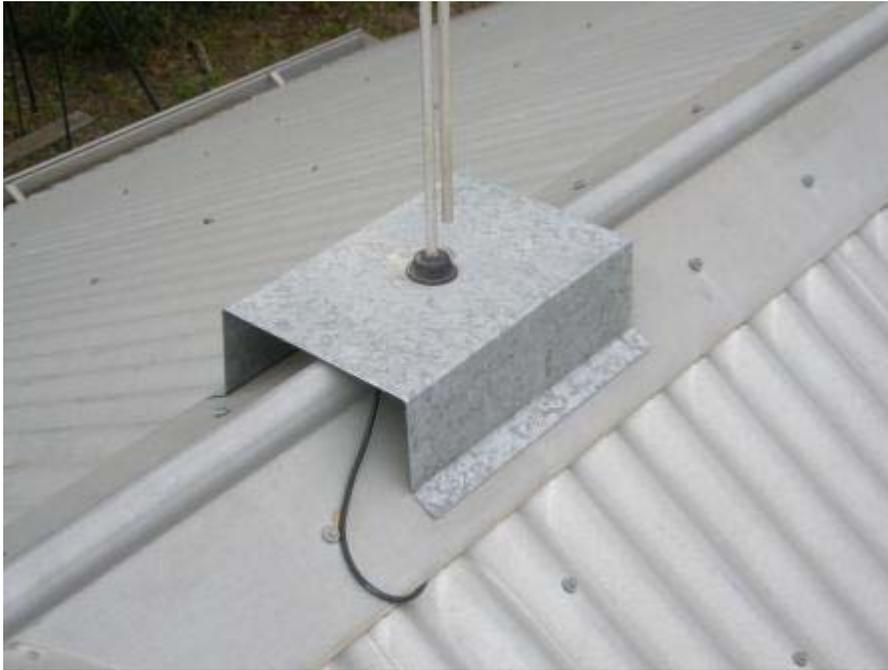
Roof mount of Shane VK3FSRG, held in place by six 3mm pop rivets.
