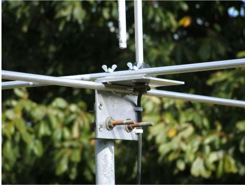
A close up shows the mounting arrangement of the two ground radials bolted to a piece of 75mm aluminium angle.
